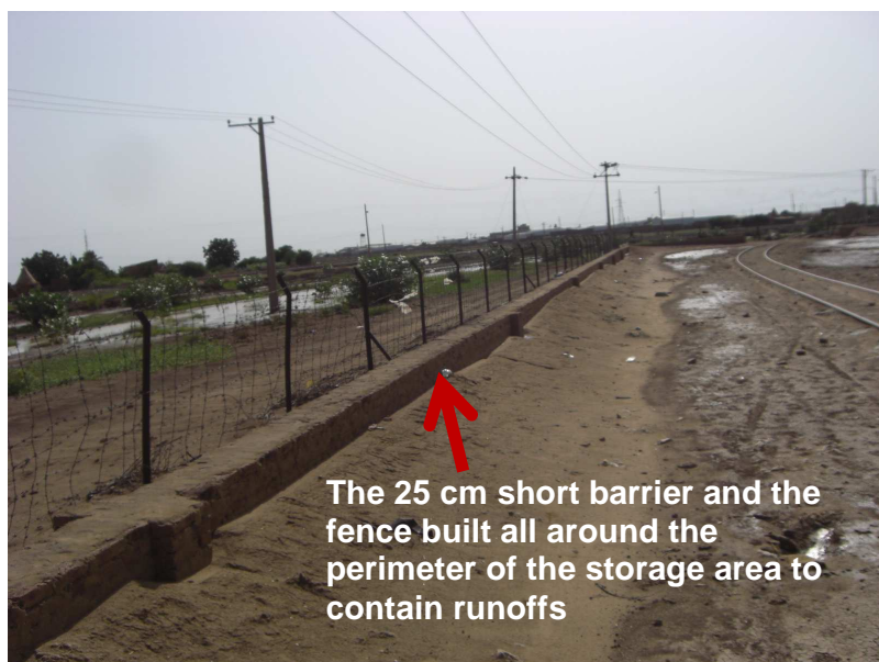
Figure S4 The fence around the perimeter of the storage, it also prevents children from entering and playing in the storage area
