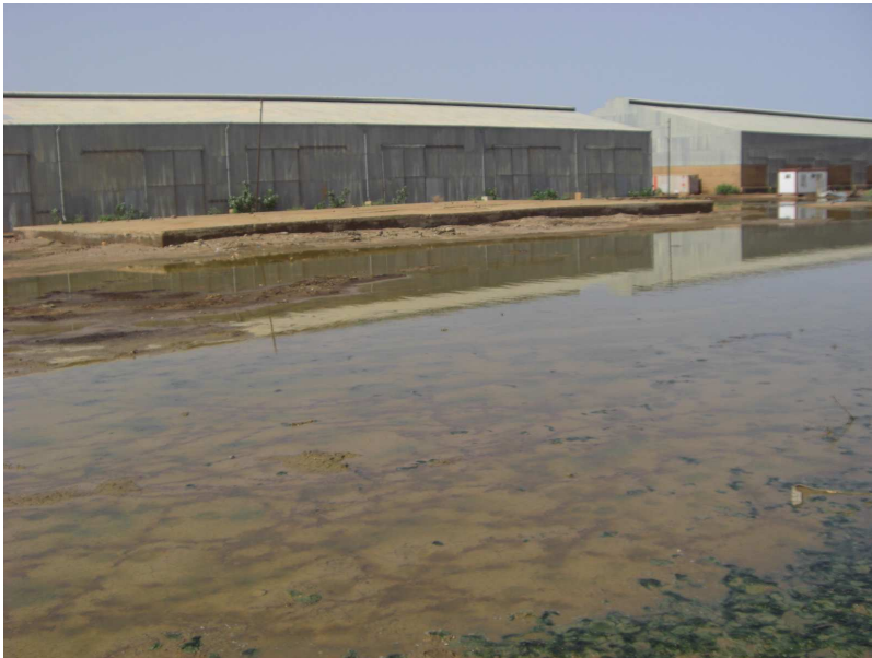
Figure S8 Containment system: the contained dump is still in good condition. Water has no colouring
