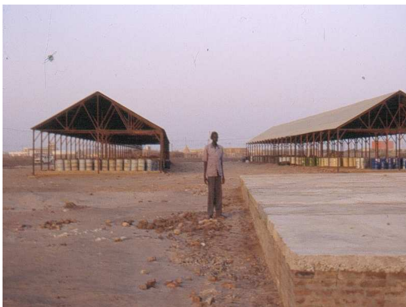
Figure S3 The pesticides grave under concrete
