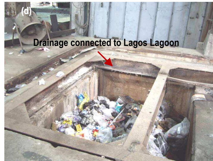
Figure N1.7 The repair shop at Site B, directly connected to the Lagos Lagoon: (a) transformers submerged in liquid, (b) transformer washing water, (c) drainage opening on the concrete slab, (d) garbage dumped into the drainage opening.
